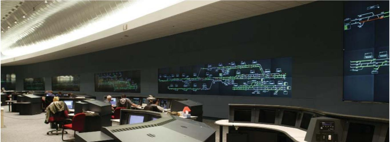
that would work with their existing network and software. A display wall consisting of 50" Mitsubishi MegaView Wall™ rear screen projection cubes, with an excellent contrast ratio and high resolution (364 pixels per sq. inch), enabled operators to see the entire rail system clearly. The wall, made up of 193 cubes and spanning an impressive 1/8th of a mile, is organized into various territory configurations.
