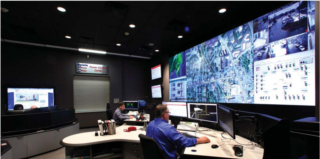
the SCADA water system. On the top right, there are nine scrolling images of the city's security cameras; on the bottom right the city's fiber loop. The four flat-panel displays allow technicians to monitor, system status, news and weather and a feed from MEAG Power, where Marietta buys its electricity. A SMART interactive touch display makes it easy to fill out and send work orders.
