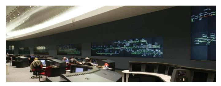
that would work with their existing network and software. A display wall consisting of 50" Mitsubishi MegaView Wall™ rear screen projection cubes, with an excellent contrast ratio and high resolution (364 pixels per sq. inch), enabled operators to see the entire rail system clearly. The wall, made up of 193 cubes and spanning an impressive 1/8th of a mile, is organized into various territory configurations.
